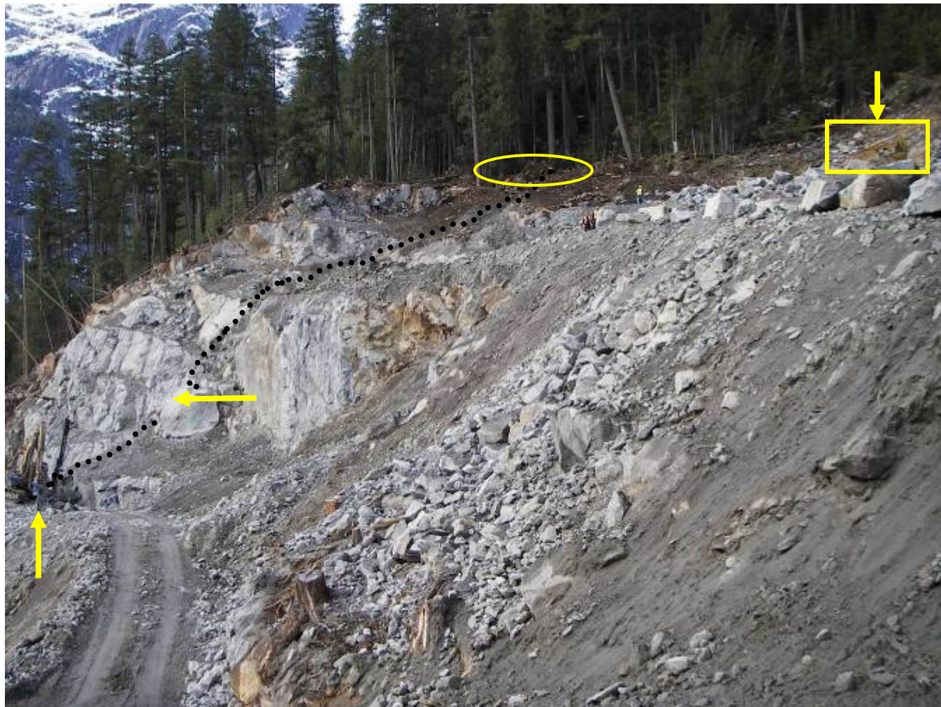
Figure 9. Overview photograph of fatal incident area. The dotted line indicates the path of the rock that the Excavator Operator and the drilling crew described. The area within the oval at the tree line is where the Excavator Operator first saw the rolling rock. The downward arrow points to the Excavator Operator's machine, which is in the area within the rectangle. The horizontal arrow points to the fatality scene. The upward arrow points to the hoe drill.
