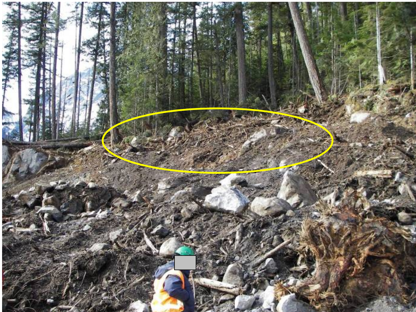
Figure 7. Rough area adjacent to previously machine-scaled ground.
