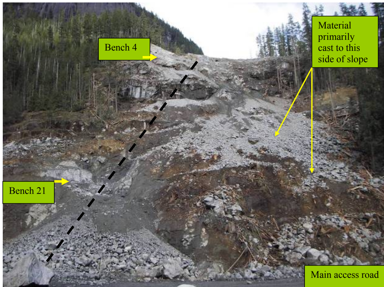
Figure 2. Mountainside at the Montrose construction site. The work at the site involved blasting and excavation to place the penstock diagonally on the slope as approximated by the dotted line.
