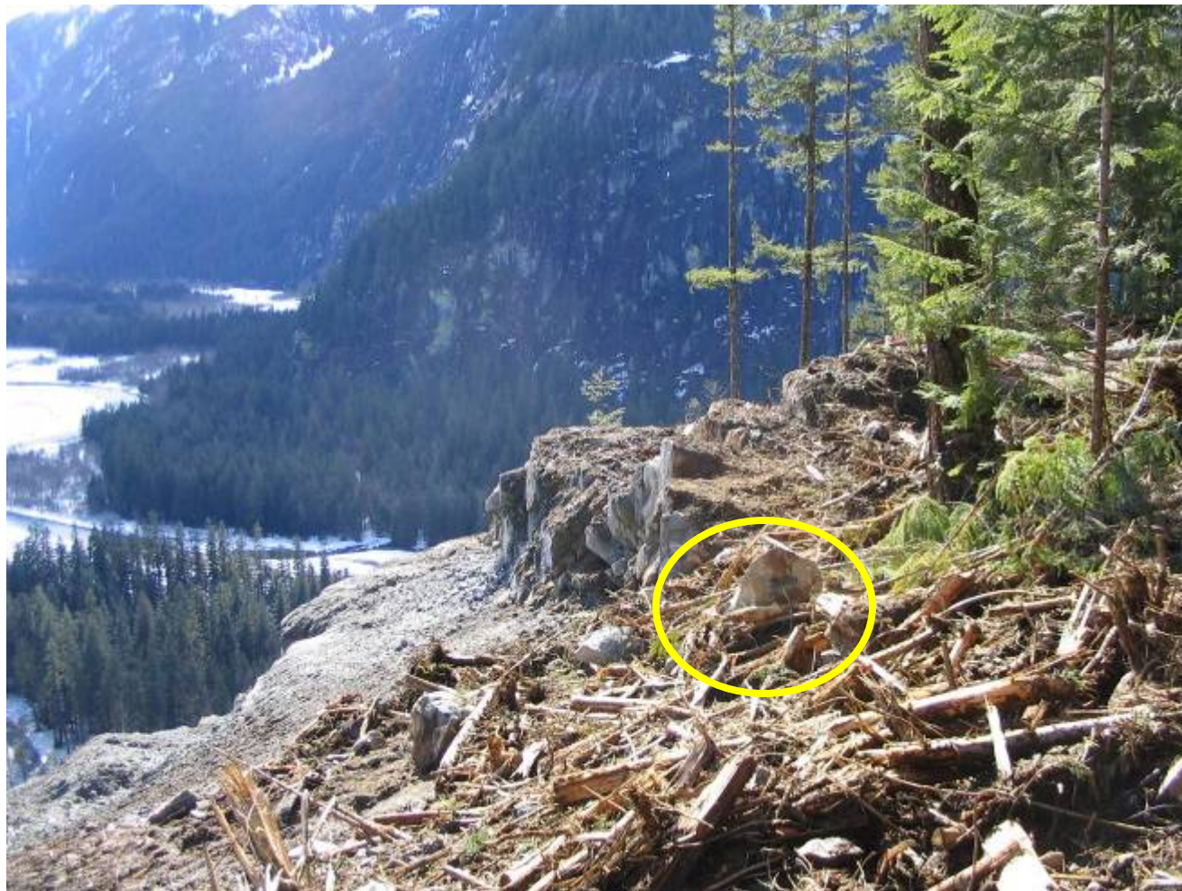
Figure 13. Unstable materials adjacent to area previously machine-scaled. A rock lying upon loose forest debris is circled.
