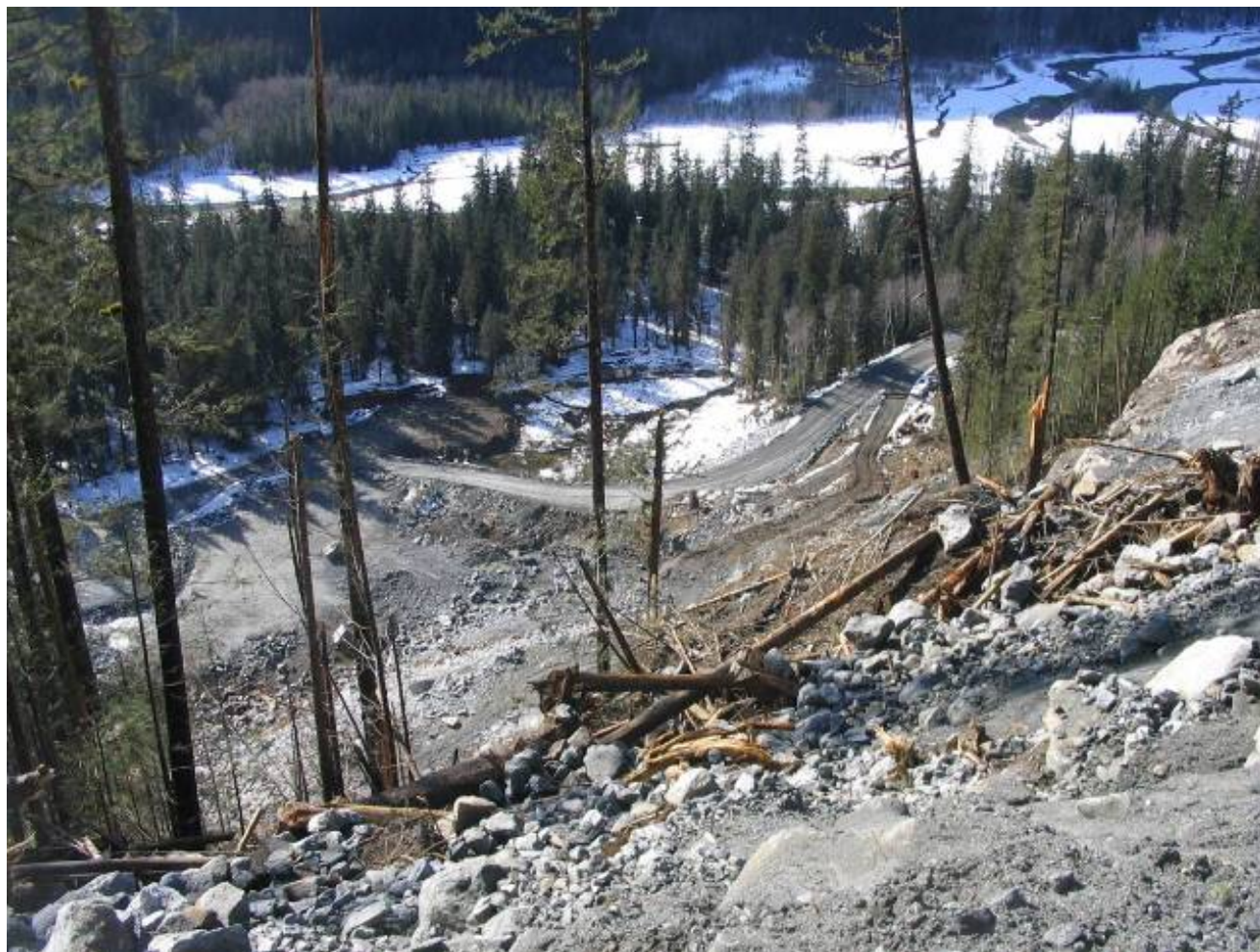
Figure 15. Unstable rock, forest debris, and logs below the Bench 4 access road and above the main access road.
