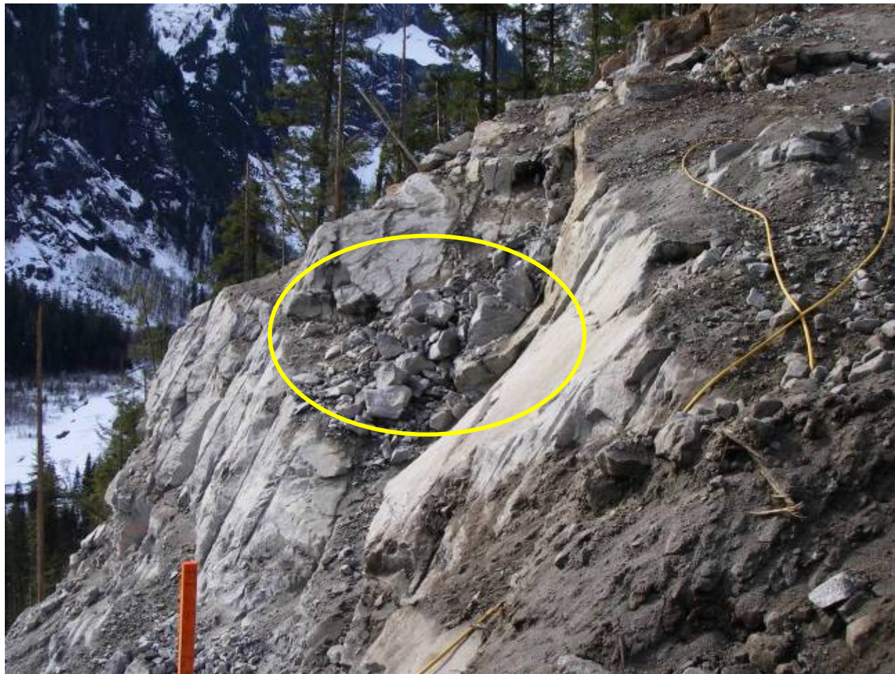
Figure 14. Loose unscaled rock above the Ranger Drill Operator's location.
