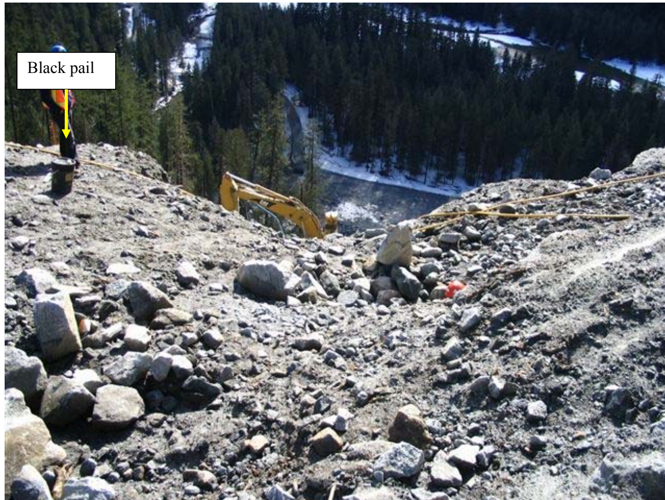
Figure 12. Trough above Bench 4. The rock rolled down the trough and beside the black pail. The upper components of the hoe drill (still where it was parked when the fatality occurred) are visible near the centre of the photograph.
