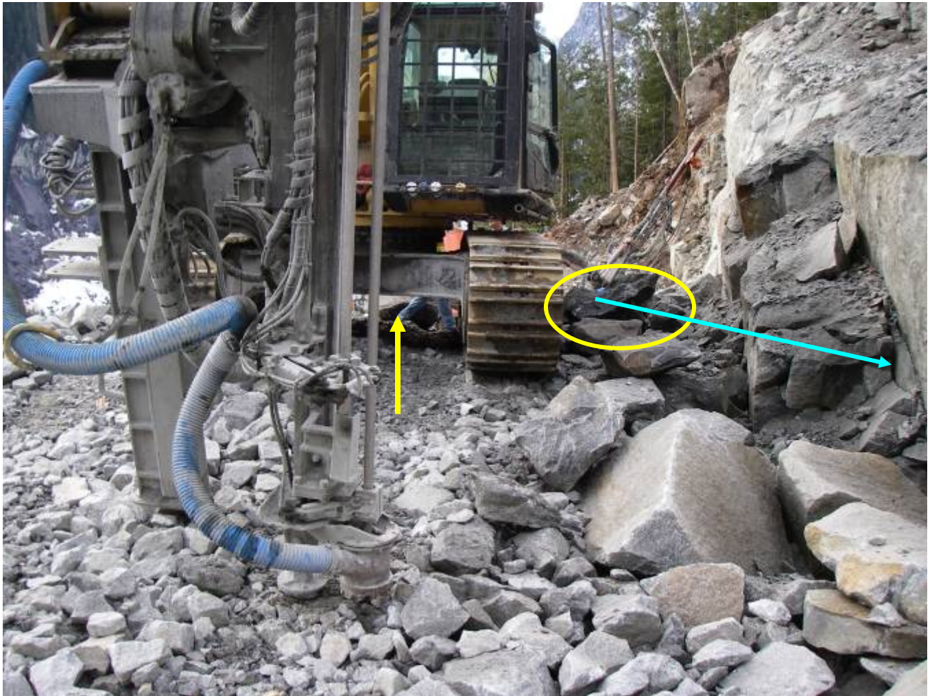
Figure 11. Rock fragments between the left track of hoe drill and the rock face are circled. The blue arrow points to where the Hoe Drill Operator moved to take shelter from the rolling rock. The yellow upward arrow points to the rock fragment behind the hoe drill.
